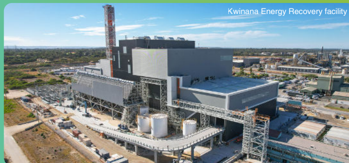
Kwinana Energy Recovery facility
